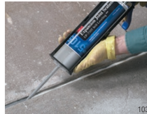
Make fast work of lengthy expansion or control joints and other larger jobs with the heavy-duty manual applicator and 12 fl. oz. duo-pak cartridges.
